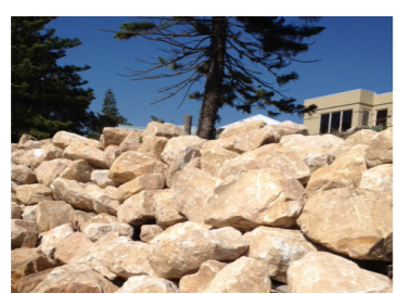
Erosion Control Sandringham
